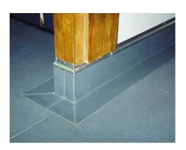
B&H COMMERCIAL SERVICES INC. HAS OBTAINED THEIR OWN CUSTOM METAL FABRICATION COMPANY. WE DESIGN ALL OUR ALUMINUM BASE CAPS, STAINLESS CORNER GUARDS AND STAINLESS DRAIN PERIMETERS TO OUR SPECIFICATIONS AS REQUIRED PER JOB SITE.
